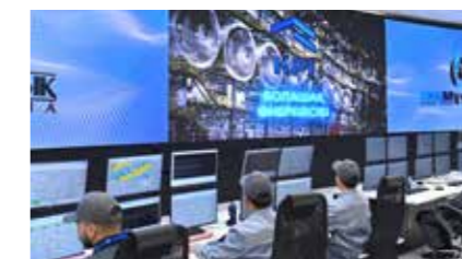
The large-scale integrated gas chemical complex of Kazakhstan Petrochemical Industries Inc. with an annual production capacity of up to 500,000 tons of polypropylene is launched.
