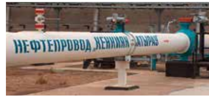
Commissioning of the Kenkiyak - Atyrau main pipeline
